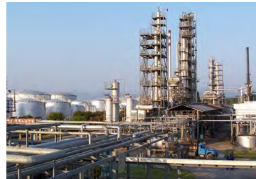
化工厂 Chemical Plant
