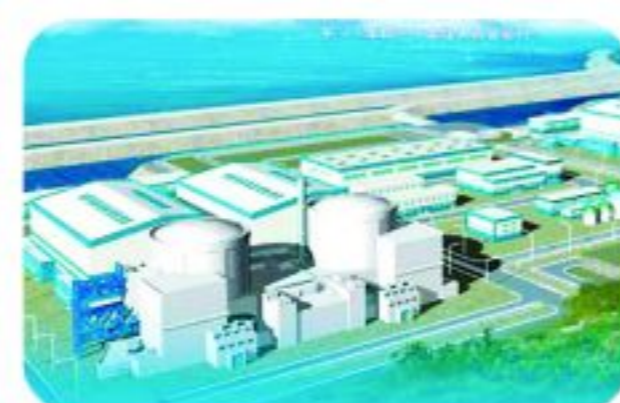
岭澳二期核电站 Ling'ao Phase II nuclear power station
