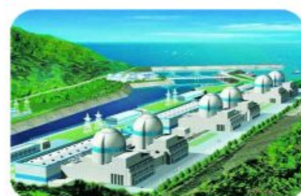
阳江核电站 Yangjiang nuclear power station
