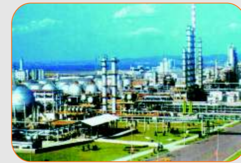
化工厂 Chemical plant
